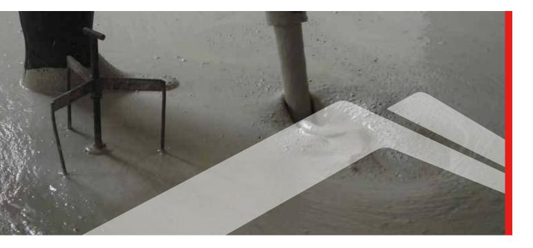
Gypsol Classic self compacting flowing screed is made to exacting standards by quality assured manufacturers to BS EN 13813:2002. It is a combination of high quality Gypsol binder, specially selected sands, water and special additives where required.
